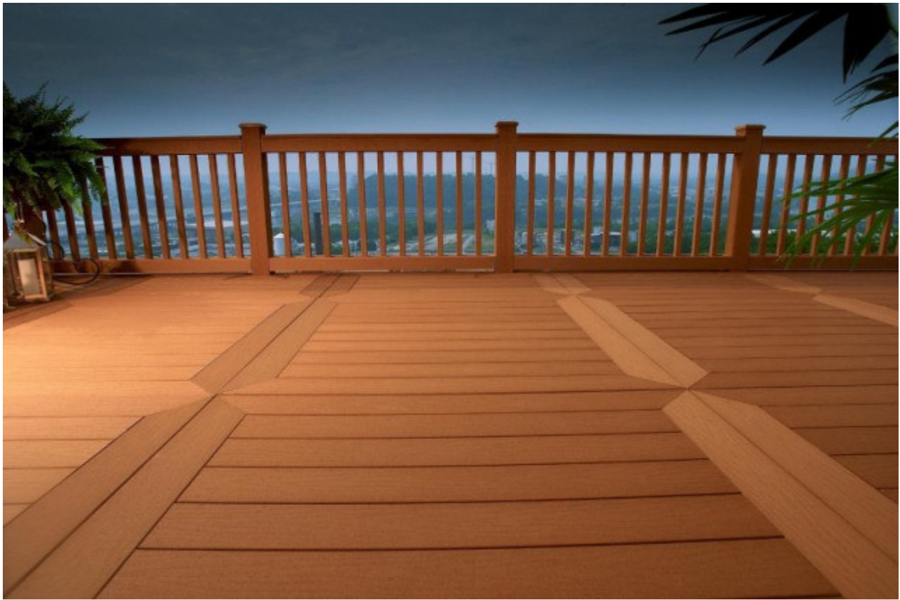
Photo of installed decking
